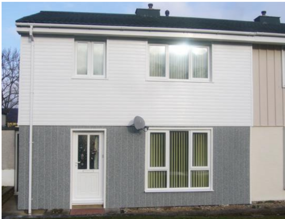
External wall insulation of a rural home in West Somerset, Sedgemoor and Taunton Deane council areas, funded by the local authorities and managed by the Centre for Sustainable Energy, saving up to 2 tonnes of CO 2 per year http://www.cse.org.uk/projects/view/1154
